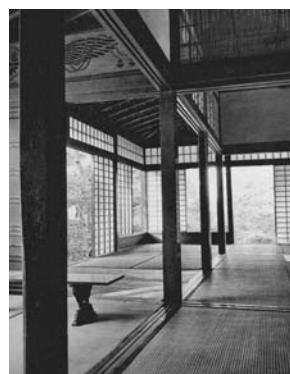
The Two Types of Sliding Doors in a Traditional Japanese House: (Top) the opaque fusuma that serve as interior partitions; (Bottom) the translucent shoji that separate indoors from outdoors. The doors slide back and forth in matching tracks mounted above on the beams and below on the floors or they can be removed completely and stored, all in response to seasons or family needs. (Photographs by Yukio Futagawa in The Essential Japanese House by Futagawa and Itoh. Chapter 10, plate 6, and Chapter 4, plate 21.)
